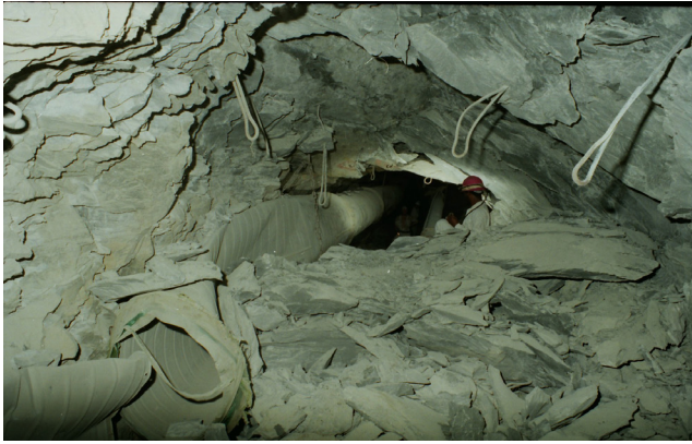
Figure 1. Damage to underground workings from a rock burst event. Source: ACG/David Ortlepp.
