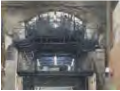
1 Metro Tunnel Project Melbourne, Australia
