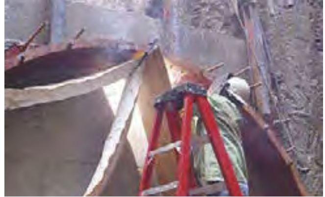
2. Welding of bolts/studs onto the sealing holder Note: BULLFLEX® hoses must be protected against sparks and molten steel
