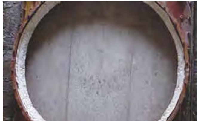
4. Fixation of the BULLFLEX® o-ring sealing in the lower area
