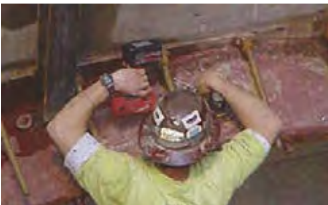
5. Fixation of filling pipes into the BULLFLEX® filling valves
