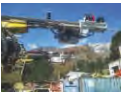
5 Rohtang Tunnel Himachal Pradesh, India
