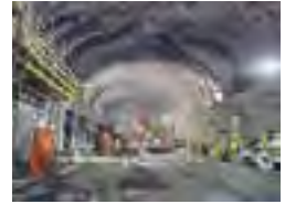
30 Alto Maipo Hydroelectric Power Plant Maipo Valley, Chile
