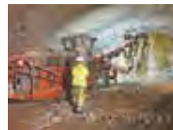
16 A26 Motorway Linz, Austria
