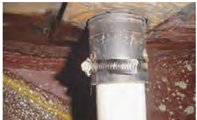
6. To be able to ensure a proper grouting sequence, filling pipes should be marked with different colors
