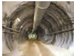
12 Tysons Corner, Dulles Corridor Metrorail Project Vienna, VA, USA
