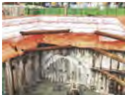
8 Eglinton Crosstown LRT Toronto, Canada
