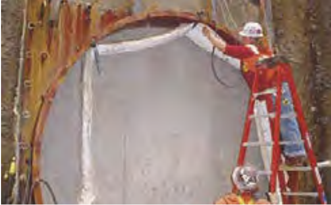
1. Mounting of the BULLFLEX® o-ring sealing for marking of the welding spots
