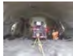
27 Tunnel Pekel Žalec, Slovenia
