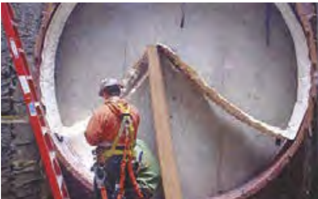
3. Fixation of the BULLFLEX® o-ring sealing in the upper area. Start of roll up with the center of the overlap at 6 o'clock position
