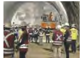
31 Extension Metro Line 3 Santiago, Chile
